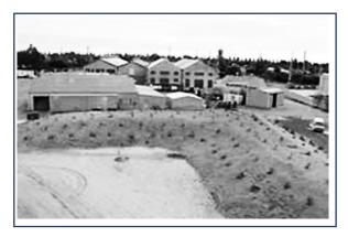
(ii) Biopile (biocells, bioheaps, biomounds, and compost piles) - Here piles of soil are placed over top of a vacuum pump which pulls air through the pile of soil to allow oxygen to get thought the soil through aeration process to the micoorganisms. Microbial activity results in the breakdown of the petroleum constituents in the soil. Biopiles are aerated most often by forcing air to move by injection or extraction through slotted or perforated piping placed throughout the pile [16].
